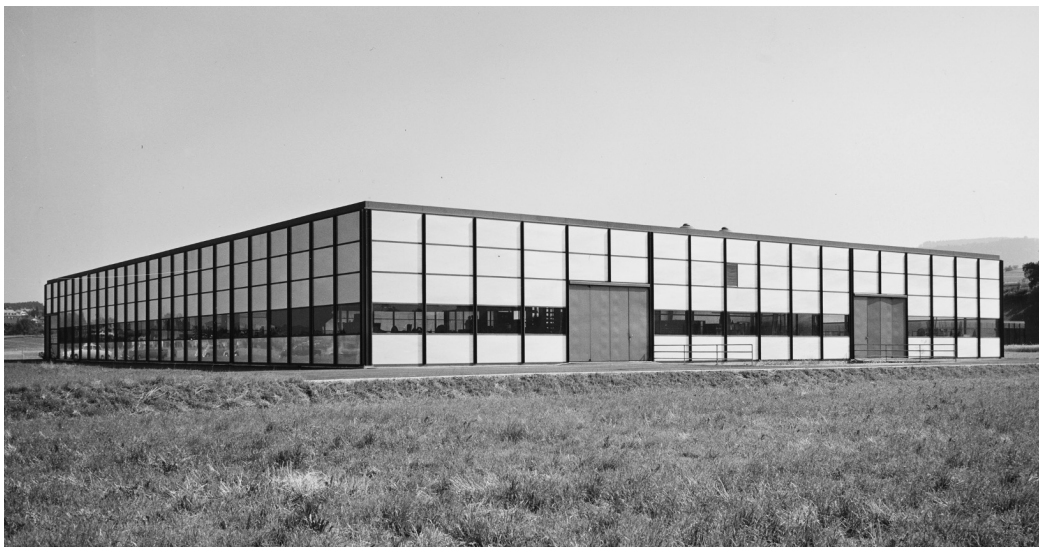
USM factory designed as a modular construction system by Fritz Haller, Münsingen/Bern, Switzerland, 1965, Fritz-Haller Archive, gta/ETH Zurich
